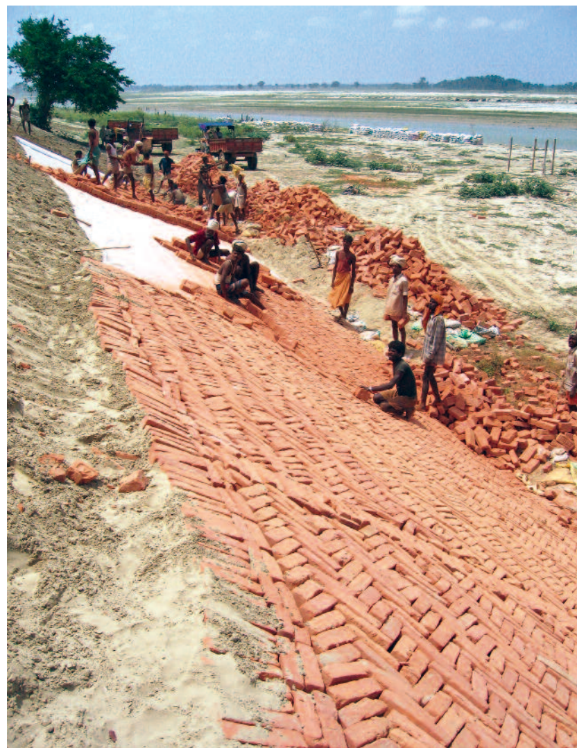
An embankment under construction
