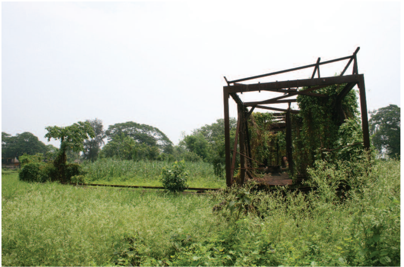
An abandoned mechanised sewage treatment plant.
